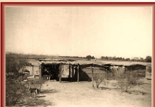
Typical home in Yoem Village, Marana, Arizona, 1936 Homes were built with railroad ties, saguaro cactus ribs, and mud, with sheet metal roofing. R. B. Spicer photo courtesy of Felipe Molina
