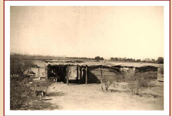
Typical home in Yoem Village, Marana, Arizona, 1936 Homes were built with railroad ties, saguaro cactus ribs, and mud, with sheet metal roofing.
