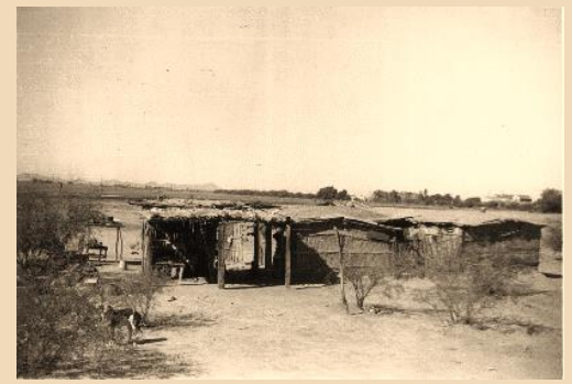
Typical home in Yoem Village, Marana, Arizona, 1936 Homes were built with railroad ties, saguaro cactus ribs, and mud, with sheet metal roofing. R. B. Spicer photo courtesy of Felipe Molina
