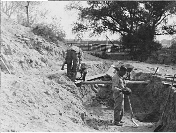
1929-1934 era photo looking east at two men excavating a test trench and a cleared area at south end of the Pueblo Grande platform mound; Tovrea cattle stockyards in background
