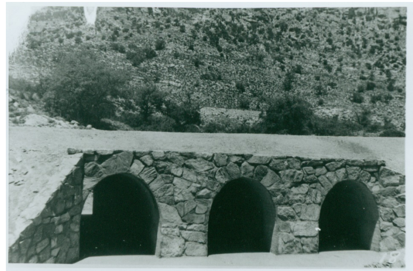
Example of prisoners' workmanship at a Catalina Highway drainage feature (Coronado National Forest photo)
