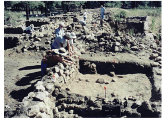
Volunteers stabilizing walls at Elden Pueblo archaeology.org
