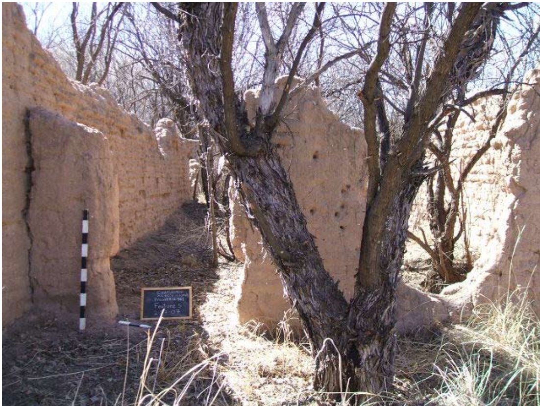
The remains of Welisch's General Merchandising. View shows the remnants of a door and a window opening. Photograph courtesy of Chris Schrager, Tucson Field Office, Bureau of Land Management.
